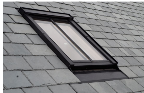
Natural slate and flush fitted rooflights
